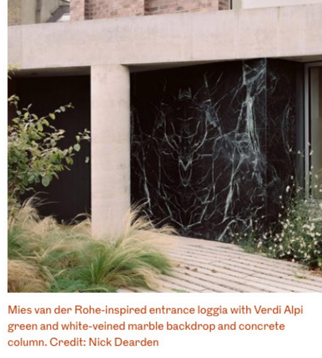
Mies van der Rohe-inspired entrance loggia with Verdi Alpi green and white-veined marble backdrop and concrete column. Credit: Nick Dearden
